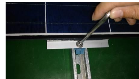
Fig.7 Installation of glass photovoltaic module
