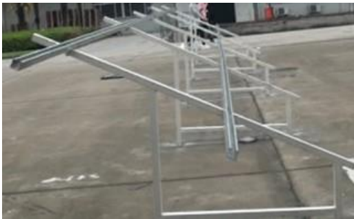
Fig.17 The bracket after be installed
