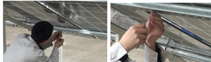
Fig. 18 Installation of glass photovoltaic module
